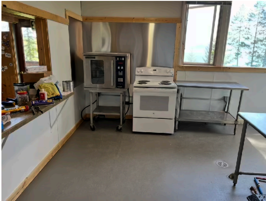
#3 KITCHEN REMODEL NEARS COMPLETION, LOOKING EAST
