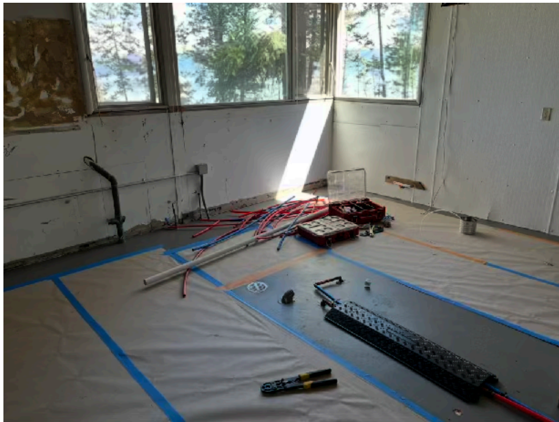
EXCITING CHANGES #1 -- LAKE LODGE KITCHEN REMODEL IN PROGRESS
