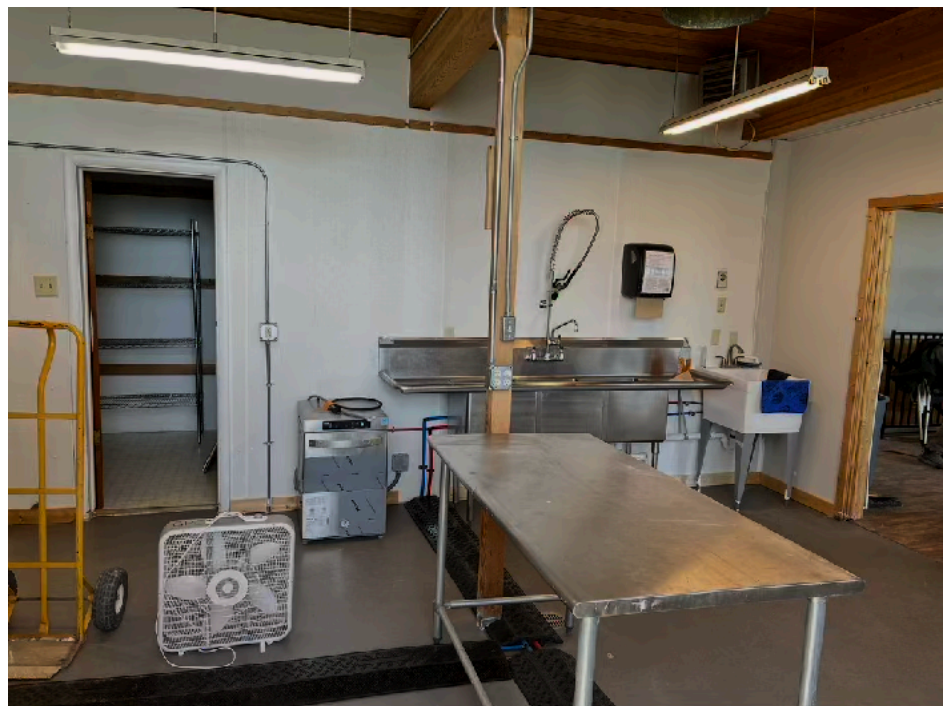
#2 KITCHEN REMODEL NEARS COMPLETION, LOOKING WEST
